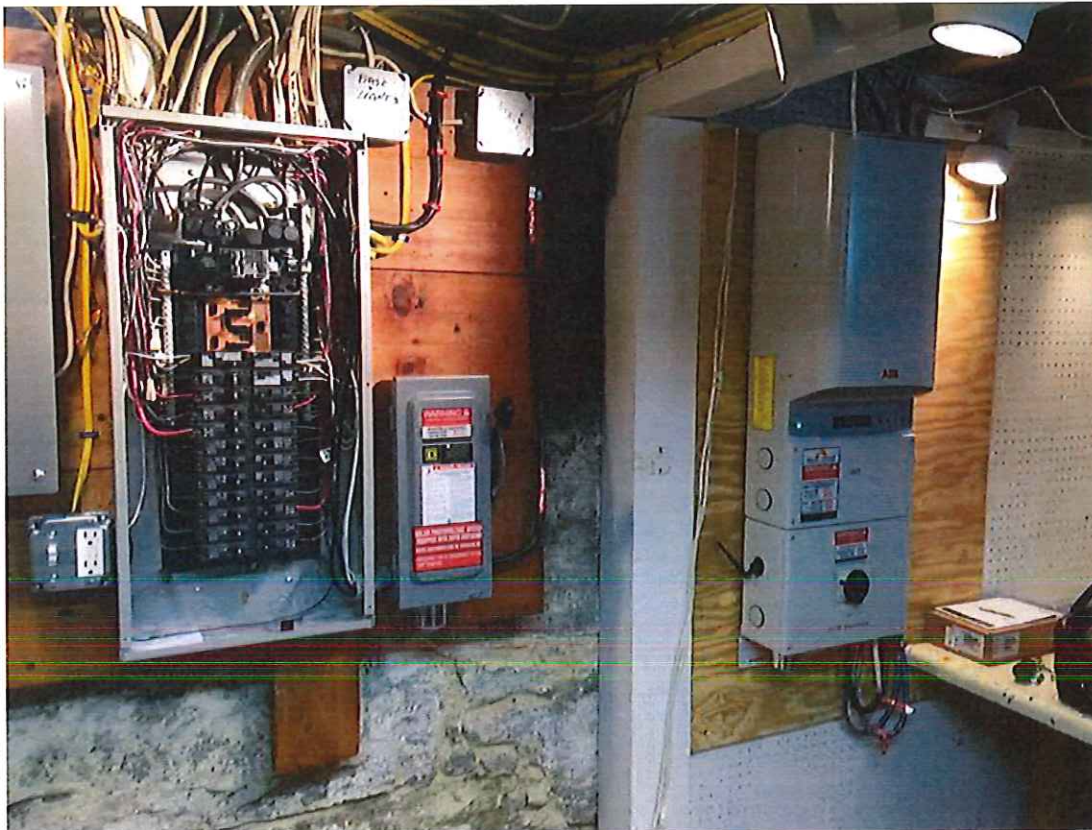
2- Point of Interconnection, AC Disconnect and Inverter
