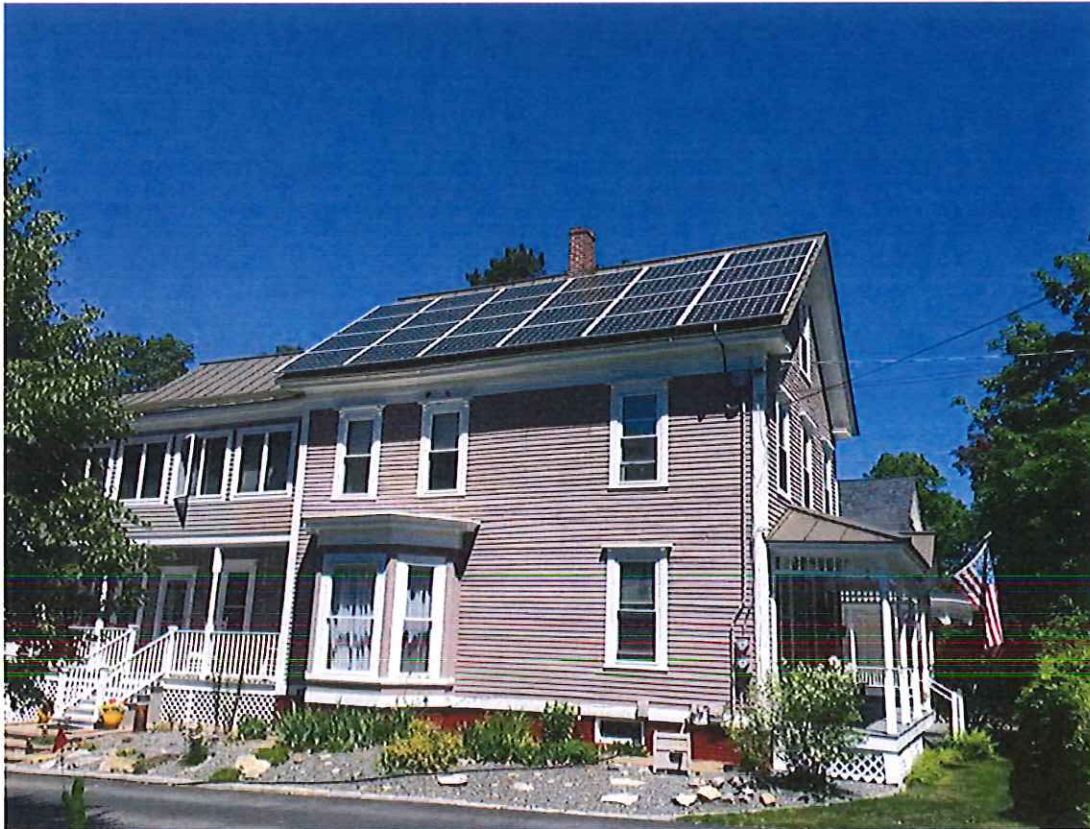
1- Completed roof mounted PV Array
